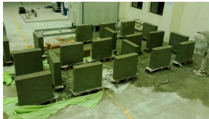
Figure 4. Masonry wallets after plastering.
