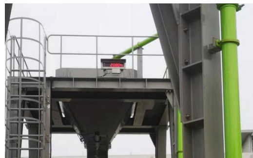
Figure 9. Concrete pumping test.
