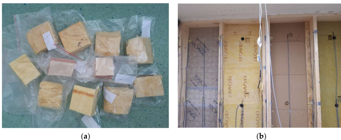
Figure 4. Process of wall disassembly (a) Part of samples collected from southern wall; (b) Photo of the eastern wall during the disassembly.
