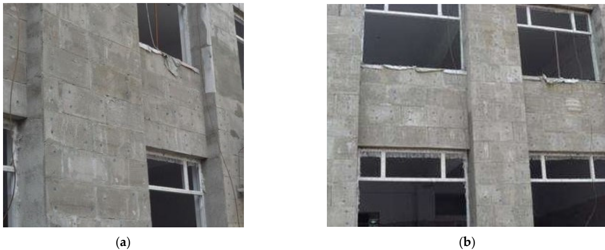
Figure 15. Building #1 exterior insulated wall panel: (a) Side view; (b) Front view.
