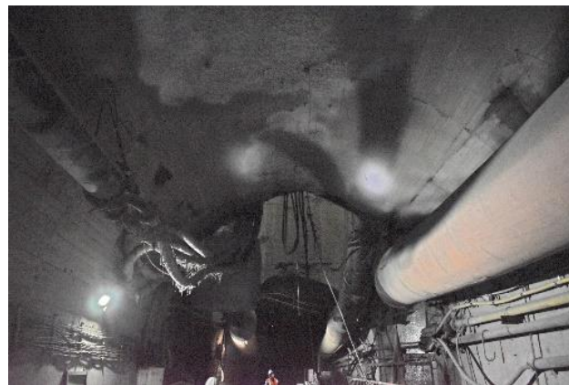
Figure 21. Maintenance of the horsehead roadway.
