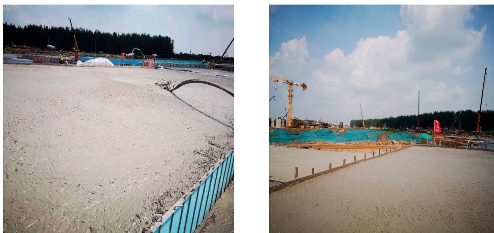
Figure 1. Pouring of FLS for intelligent networked vehicle testing site.
