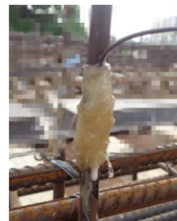
(b) Strain gauge installation
