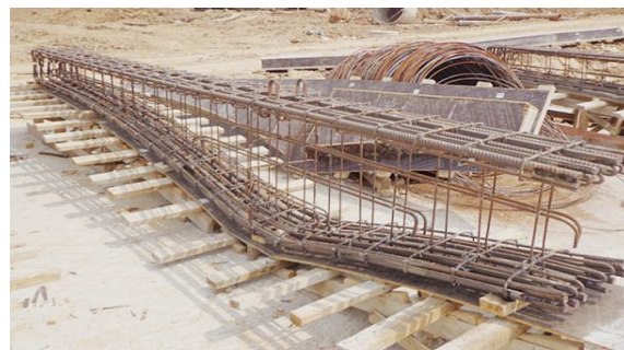
(a) Rebar binding
