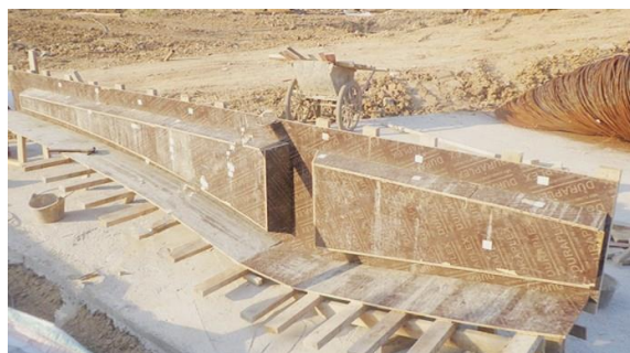
(c) Formwork assembling
