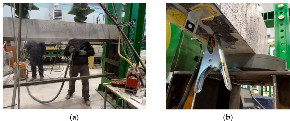
**Figure 10.** The process of strengthening reinforced concrete beams: (a) Making a groove from the bottom surface of the beams; (b) View of the copper flat bar with the current wire connected [33].
