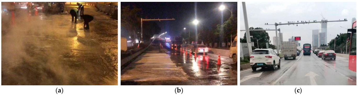
Figure 2. Applications of rapid-hardening HSFRC in practices. (a) Casting of concrete. (b) Hardening of concrete. (c) Operation situation for 3 years.
