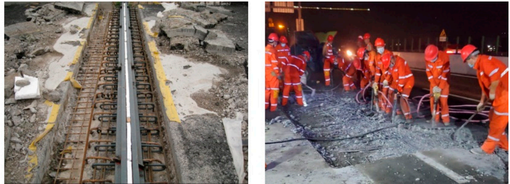
Figure 1. Expansion joints and corresponding repair work in bridge engineering.
