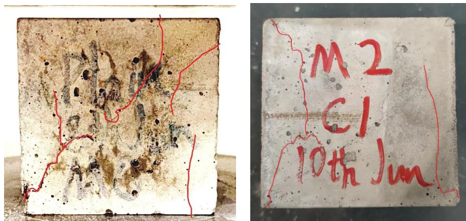
Figure 3. Cracks of the specimen after the compression test by contrast. (Left is cube of M_0 , and right is cube of M_2 ).
