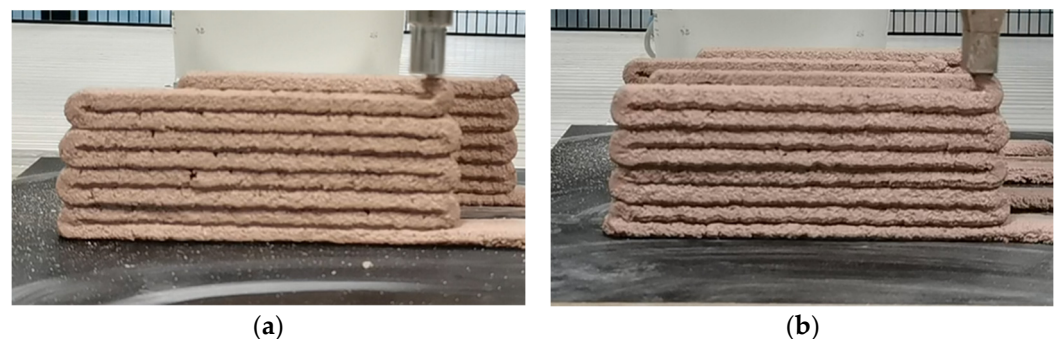
Figure 3. The influence of the nozzle section on the micro-cracking during the printing of clay-gypsum-pozzolan mortar: (a) round cross-section; (b) square cross-section.
