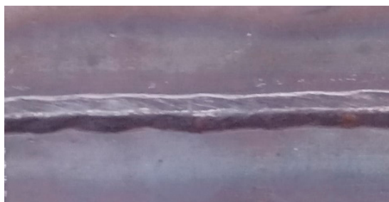
Figure 3. Single-pass weld joint obtained by MAG (Metal Active Gas) process with X16 wire.
