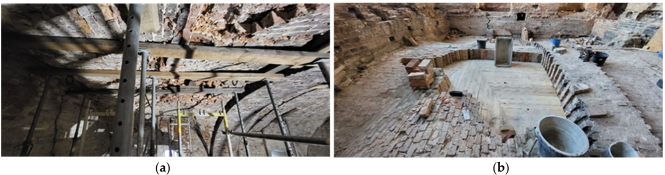
Figure 16. Fragments of the vaults above the ground floor of the castle: (a) view of the damaged bricks from below; (b) filling in (photos by authors).
