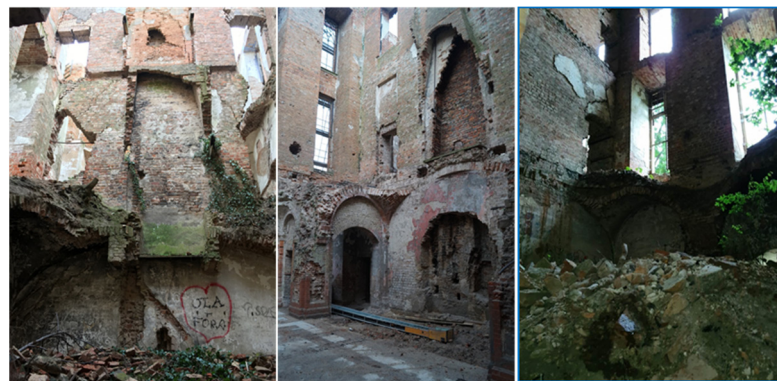
Figure 2. View of walls and vaults—as of 2018 (photos by authors).
