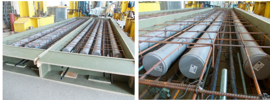
Figure 7. The sample slabs before concreting.
