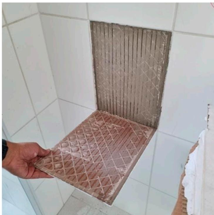
**Figure 2.** Detail of the ceramic tile detached from the adhesive mortar.
