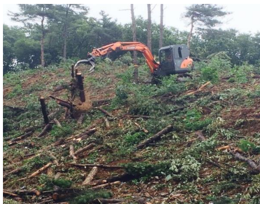
Figure 1. Log extraction using a small shovel-mounted steel-track excavator with a log grapple (1.3 m maximum jaw opening and 0.1 m closed jar gap); the boom length of the excavator is 5.1 m (Photo create: E. Lee).
