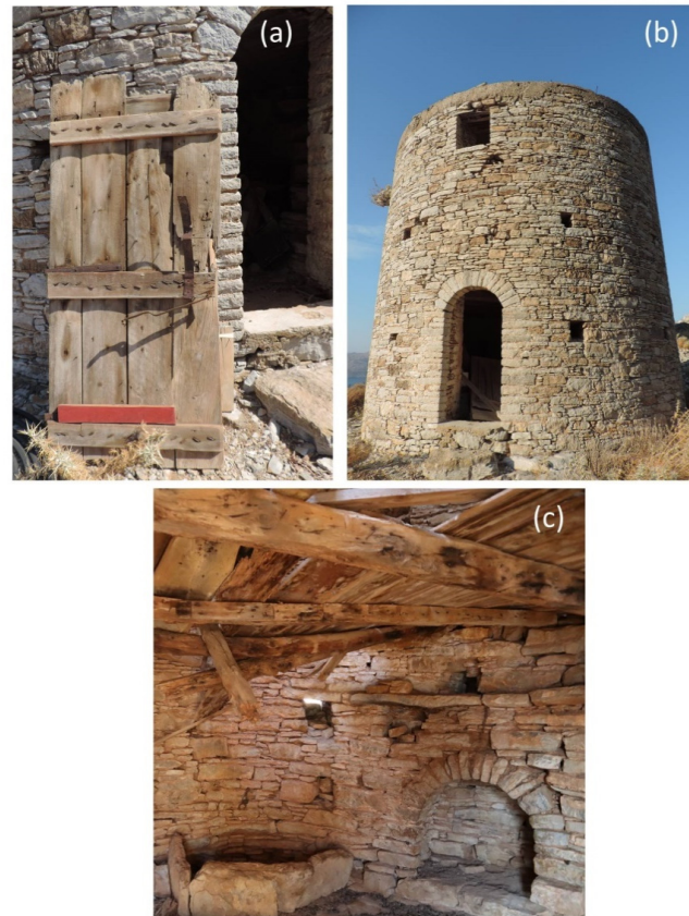
Figure 2. Historical timber examined in the current study: (a) one of the examined doors; (b) one of the standing windmills on a hill to the east of Ano Symi; (c) its interior.
