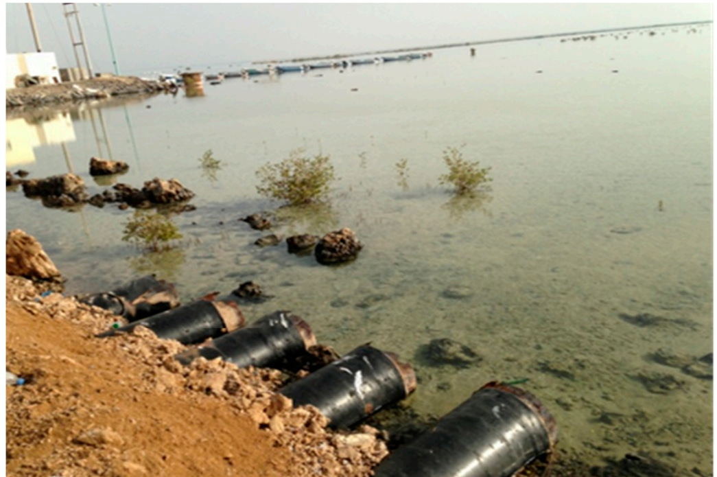
Figure 12. Pipes laid down under the sand passage to allow water circulation.
