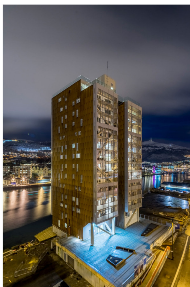
Figure 5. Treet—timber tower apartment building in Bergen, Photograph by David Valideby [52].
