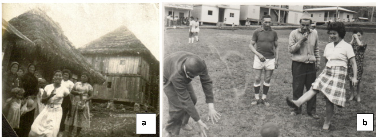
Figure 6. Women have been present in formalizing and promoting conservation programs and other sustainable development ventures in the area. The left picture (a) shows the original wooden structures with thatch roof, while on the right (b) the houses are already brick with metal roofs. Source (a) from Jack Rodríguez, Mar 1952. Source (b) from Jack Rodríguez, May September 1988.
