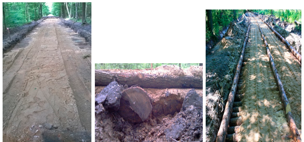
Figure 1. Reinforcement of the roadbed in the studied sections—oak and pine logs.
