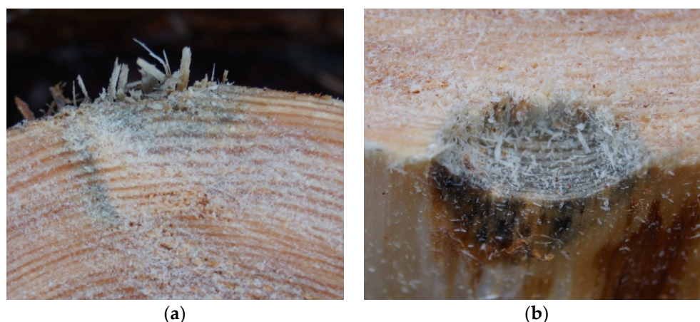
Figure 3. (a,b) Blue stain in damaged zones.
