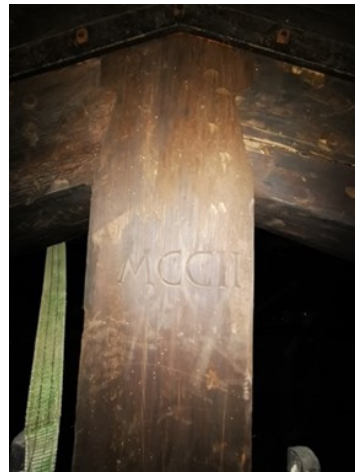
Figure 8. One of the elm wood king posts of the central nave shows a graved possible dating (MCCII). In this case, the graved year would be more than two centuries before the assembling of the roof, marking a possible reuse from a previous structure.
