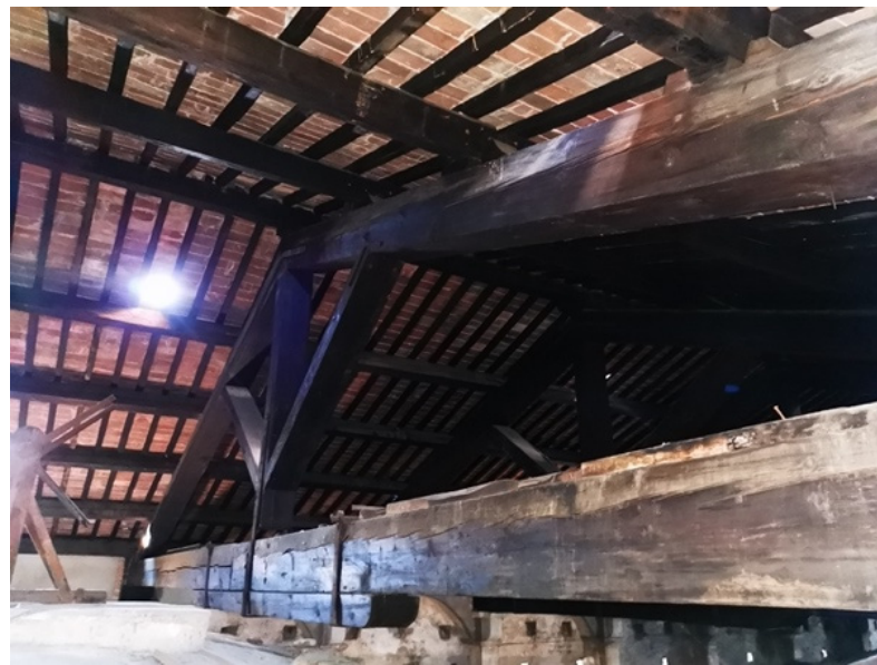
Figure 2. One of the trusses of the central nave.
