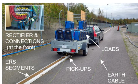
Figure 2. Experimental setup at the Elonroad pilot test site.
