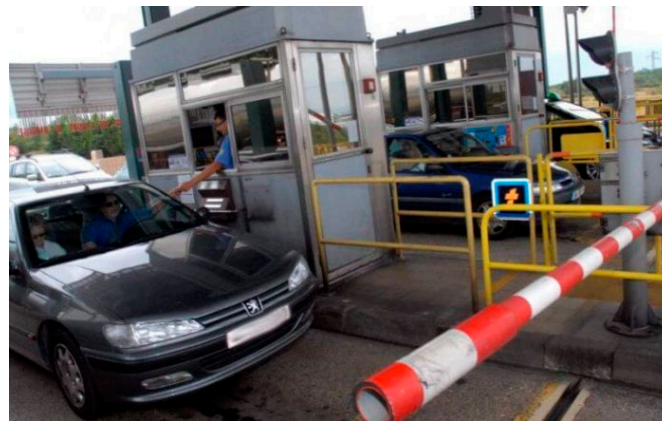
Figure 5. Example of entry and exit gates of a DWCS road.
