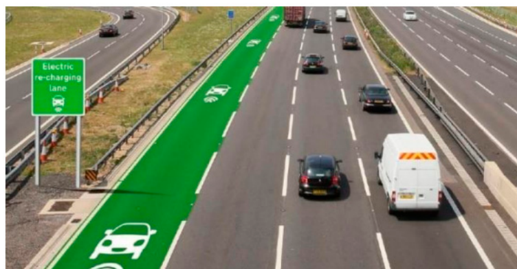
Figure 2. Highway with a DWCS.
