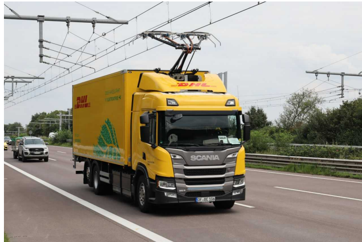
Figure 8. The dynamic charging technology using an overhead contact line employed by Project FESH in Germany (reproduced with permission from FuE-Zentrum FH Kiel GmbH).
