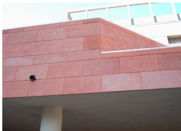
Figure 10. A detail of Teatro Massimo in Cagliari; the cladding, installed following a “run” pattern with runs in variable heights, was built using Fordongianus red “trachyte” (renewed in 2009).
