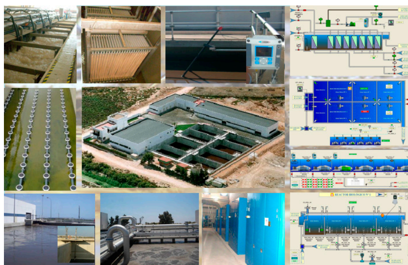
Figure 8. Aeration elements in San Pedro del Pinatar wastewater treatment plants (WWTP) with activated sludge (AS) + membrane biological reactor (MBR) technology.
