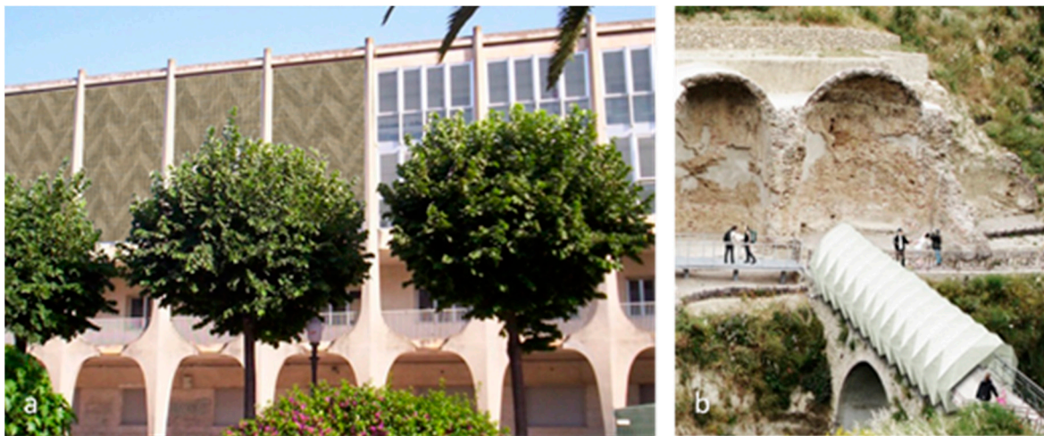
Figure 2. The novel composite material application: (a) as second skin to refurbish an existing building; (b) as temporary pavilion envelope.
