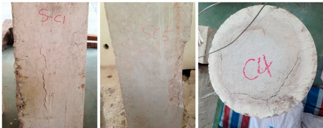
(b) crack on side
