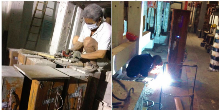
(c) Smoothing, welding
