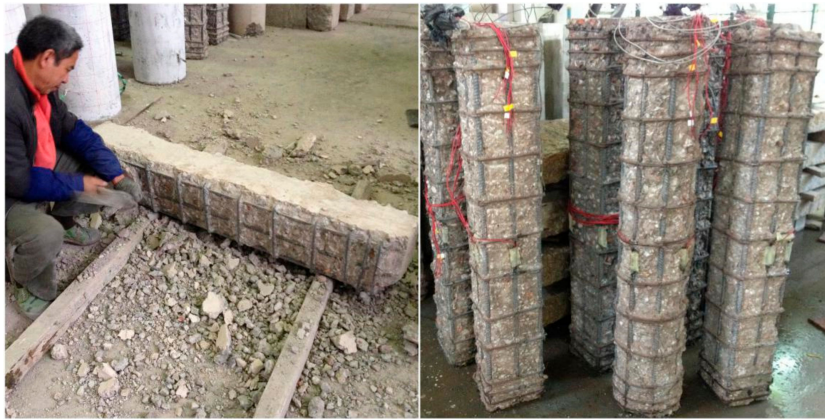
(a) removing the damaged surface, cleaning and saturating the specimens
