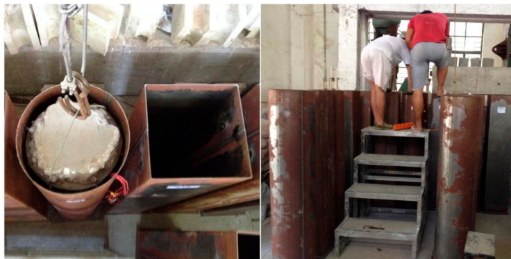
(b) wrapping steel tube, grouting
