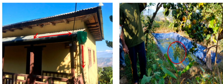
Figure 5. Roof collection system for rainwater: (a) The arrow shows the flow direction of rainwater runoff; (b) the red circle marks the rainwater reservoir.
