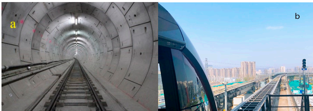
Figure 1. A track structure comparison of a metro system and an Elevated Electromagnetic Suspension (EMS) Maglev system: (a) a typical rail-track structure of a traditional metro system [17]; (b) EMS Maglev track structure of the Beijing Maglev Express.
