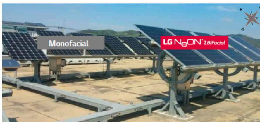
Figure 1. Monofacial and bifacial photovoltaic (PV) systems monitored for the period of June 2016–May 2017.
