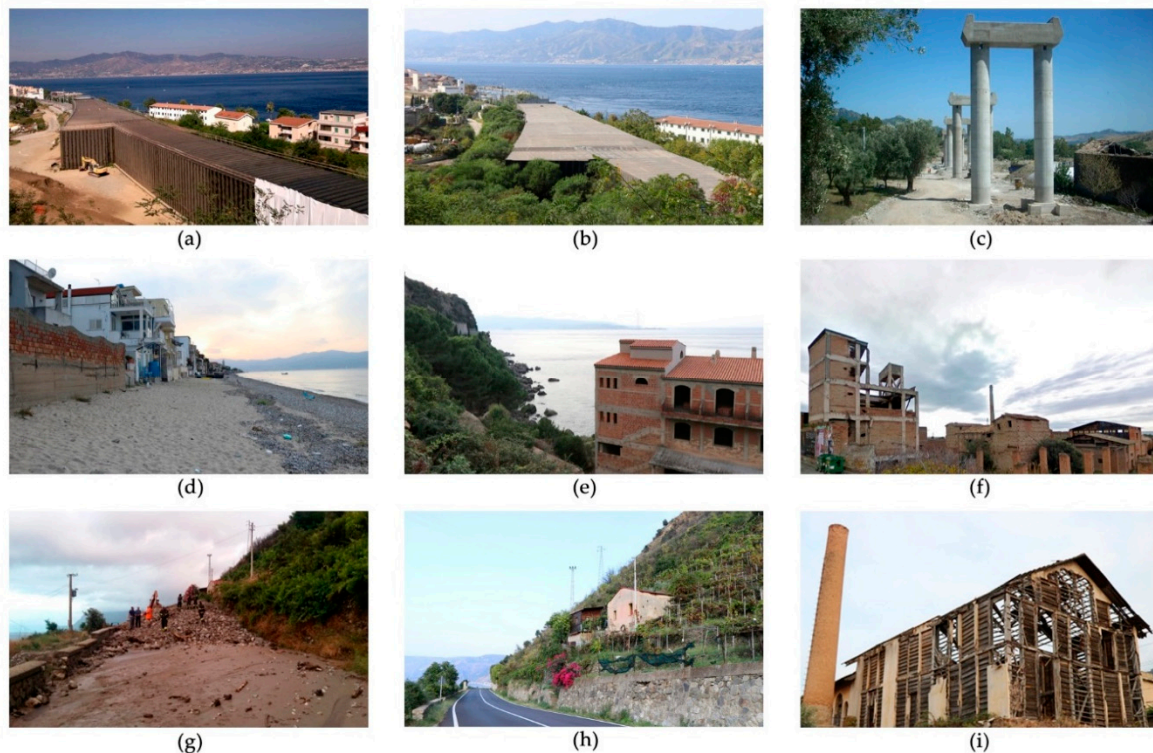
Figure 5. (a,b) Variant of the Cannitello-Villa San Giovanni railway line, preparatory work for the start of construction of the Bridge over the Strait, never built; (c) modernisation works of Bovalino-Bagnara, a transversal artery connecting the Mediterranean Motorway to the SS 106, never completed; (d,e) abusive or abandoned building near the Tyrrhenian coast; (f) Aspromonte wood processing inactive plant of the XIX century. The buildings have industrial archaeology restrictions imposed by superintendence; (g,h) a collapsed terrace due to the abandonment of crops, then recovered and recultivated; (i) abandoned spinning mill of the XIX century.
