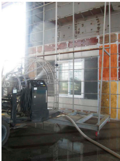
(c) Air leakage test
