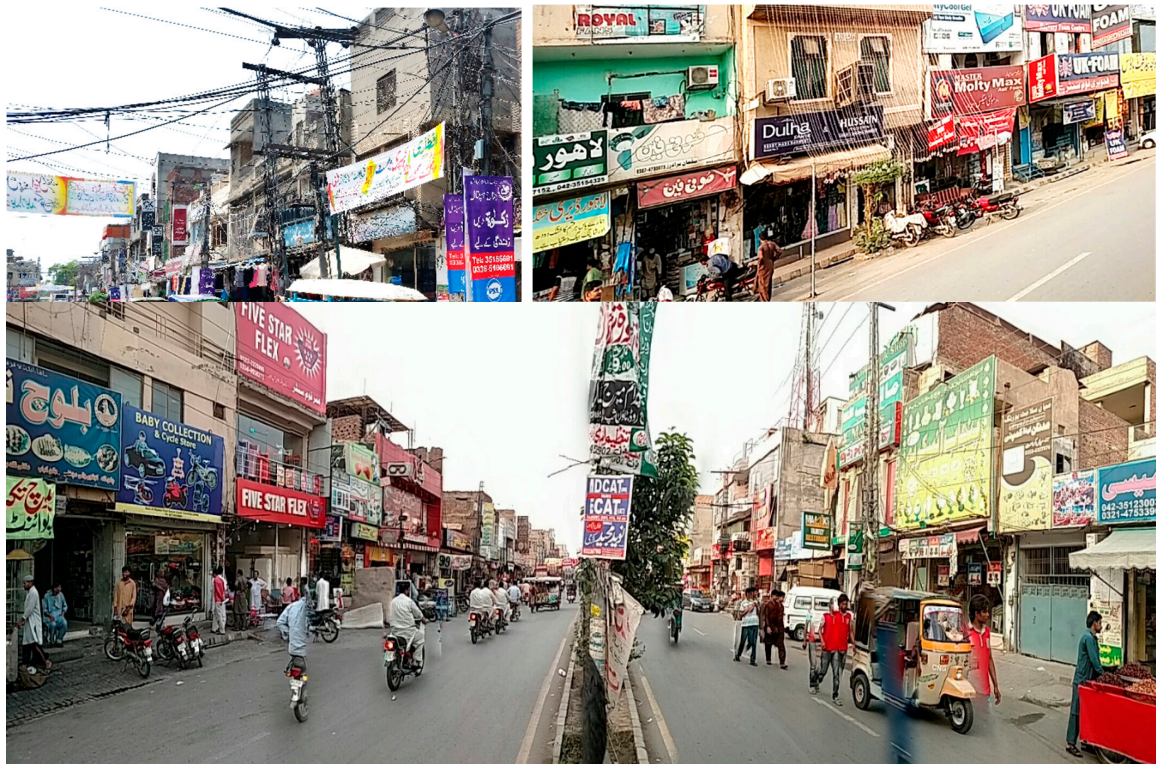
Figure 4. Pictures from the streets of Lahore, Pakistan capturing some key VPOs including outdoor advertisements, poles, hanging and cluttered wires, architecturally poor structures, dilapidated building and encroachments.
