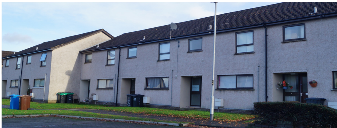
Figure 1. The 'no-fines' social houses.
