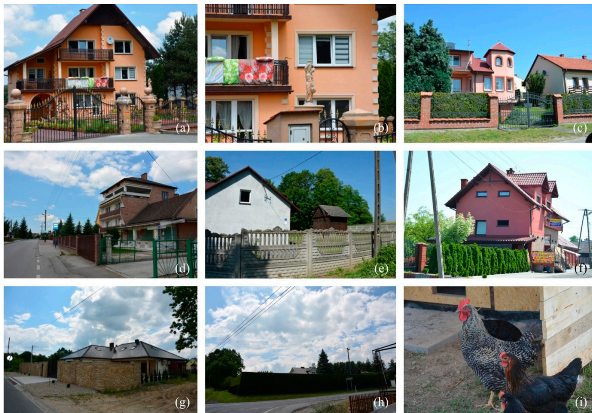
Figure 9. Processes related to the progressing semiurbanisation identified in the municipality of Skawina, part 2, (a)–(c).—Colour schemes of façades and introduction of exotic features, as identified in Wielkie Drogi and Polanka Hallera (d)–(f).—Construction dissonance as seen in Kopanka, Sosnowice, and Krzęcin, (g)–(i).—Discontinuity of relationships between rural residents and migrants from the city.
