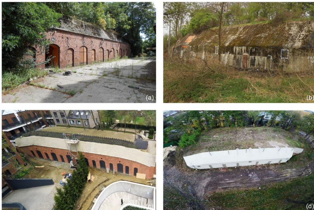
Figure 1. Examples of work that cause soil and plant ecosystem degradation of historical green roofs: (a,c) Infantry shelter before and after restoration; (b,d) infantry shelter before and during restoration works with a new green roof, Wrocław, Poland. 2012 and 2016, sourced from the author Łukasz Pardela’s archive.
