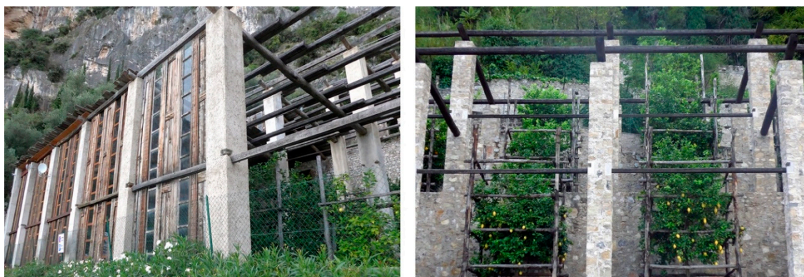
Figure 10. Lemon houses at Lake Garda; left: partly enclosed and partly open structure; right: lemon trees with scaffolding. Photography: Defne Sunguroğlu Hensel, 2019.
