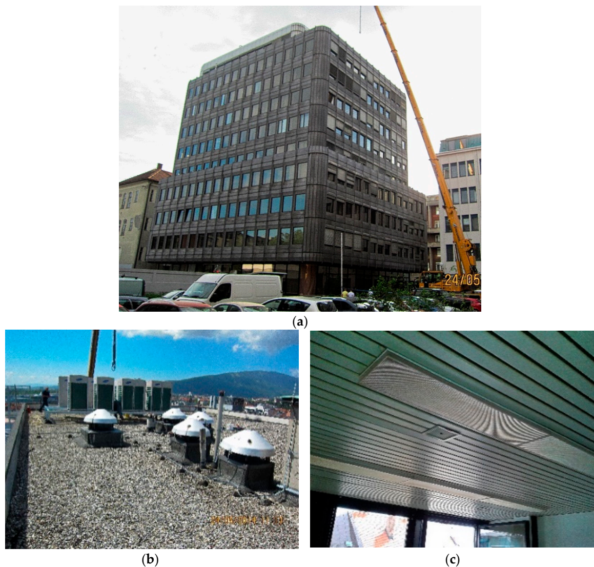
Figure 3. Office building: North and East—with exterior shades—façade (a); roof (b); lamellar lowered ceiling (c). Source: Marinič [62].
