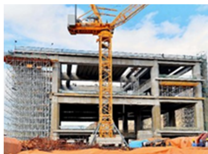
Figure 6. Construction mockup for the nonhistorical part in the workshop area.
