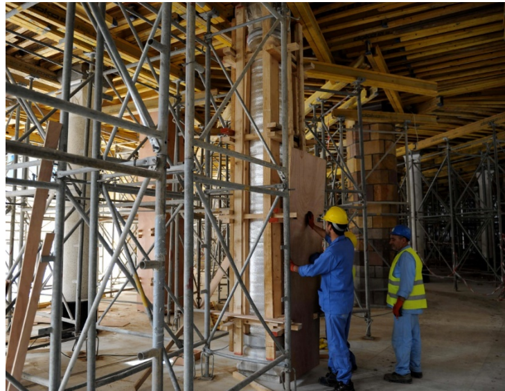
Figure 19. Protection, propping, and packaging of a historical column before dismantling.
