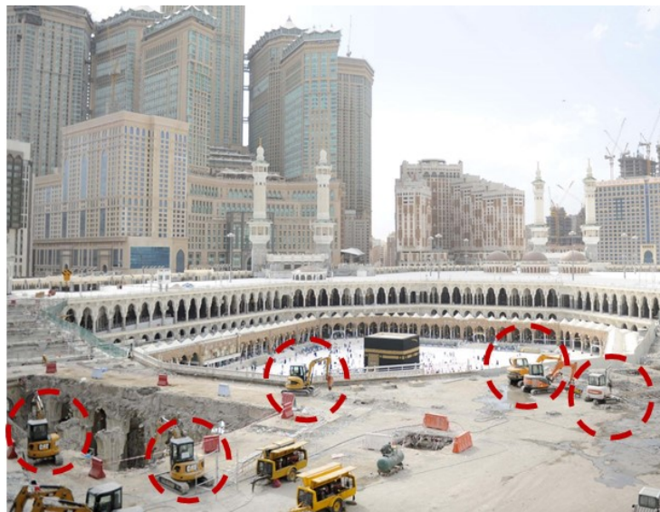
Figure 11. Small machinery (shown in the red circles) at the project site.
