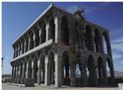
Figure 4. Demolition mockup for the nonhistorical part in the workshop area.
