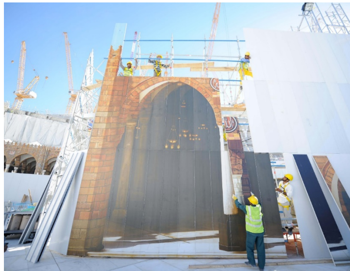
Figure 13. Temporary fences mimic the project shape.
