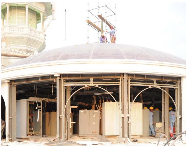
Figure 15. Rerouting work for an electrical service room.
