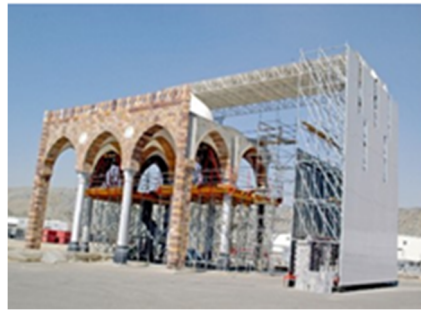
Figure 3. Demolition mockup for the historical part in the workshop area.
