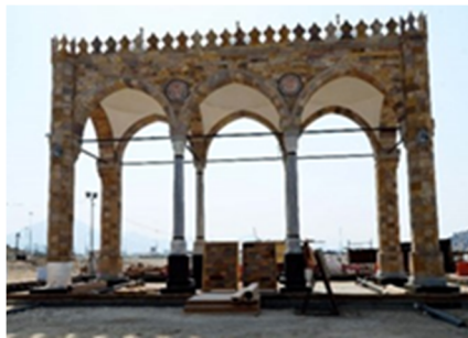
Figure 5. Construction mockup for the historical part in the workshop area.
