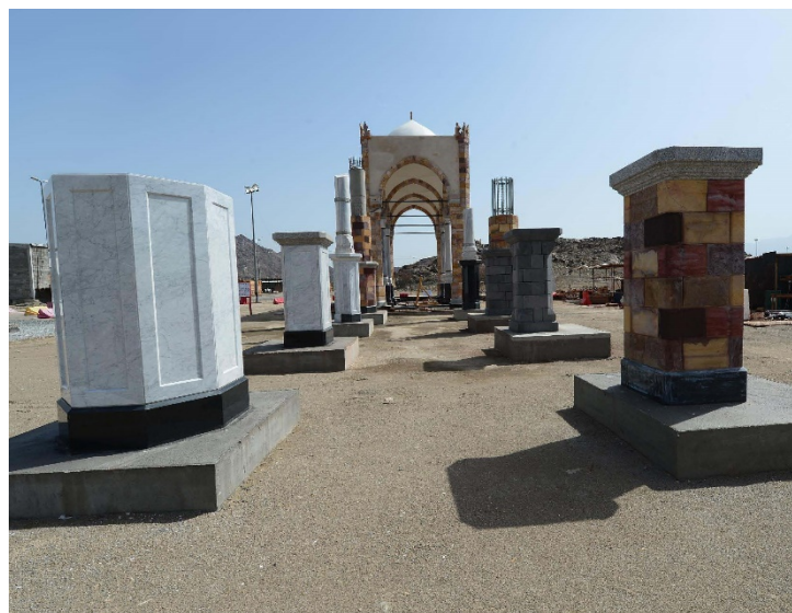
Figure 23. Columns, bases, and material mockups for the historical part.
