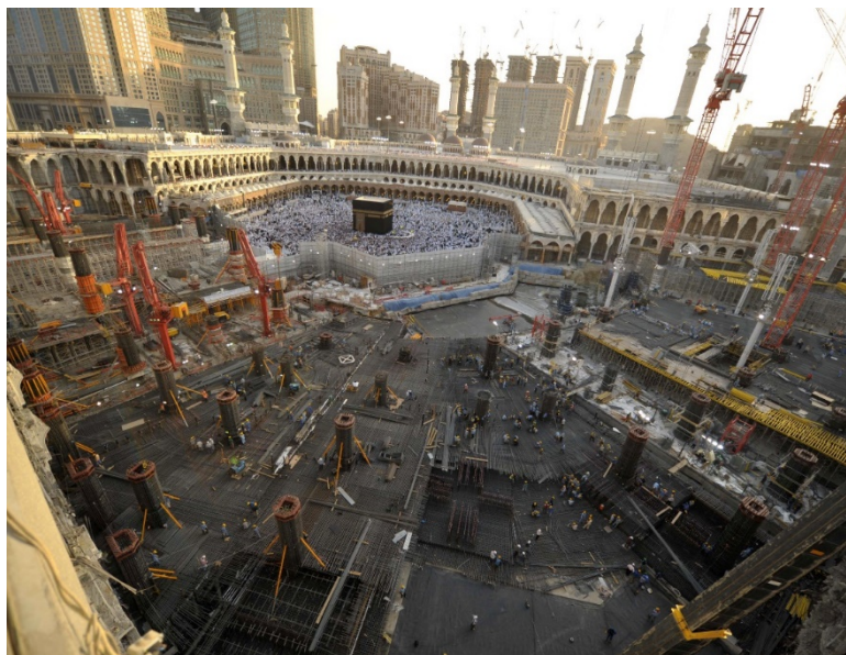
Figure 16. Steel reinforcement density in the raft foundation.
