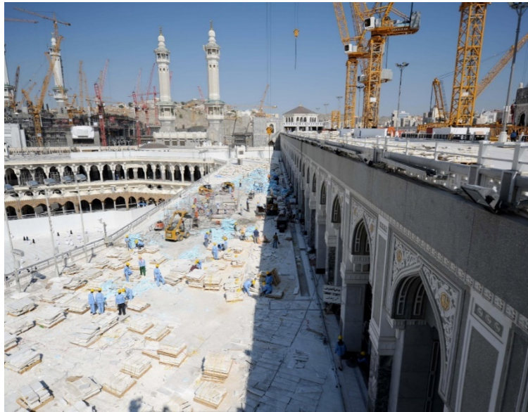
Figure 14. Marble and roofing system material removal.
