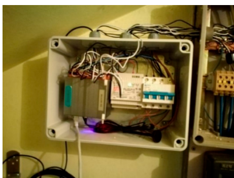
Figure 5. Installation of the datalogger (Source: Ekitermik Efizientzia Energetikoa).
