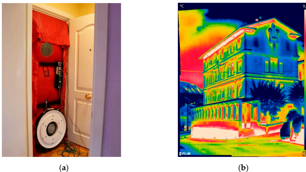
Figure 4. (a) Installation of the fan to test the permeability of the windows; (b) Thermography of the main facade. (Source: LCCE).
