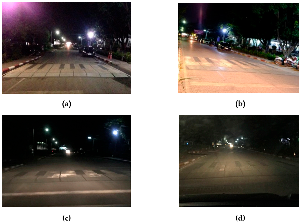
Figure 13. 3DPK crossing during nighttime showing faded paint: (a) One week after installation, (b) four weeks after installation, (c) eight weeks after installation, and (d) 12 weeks after installation.
