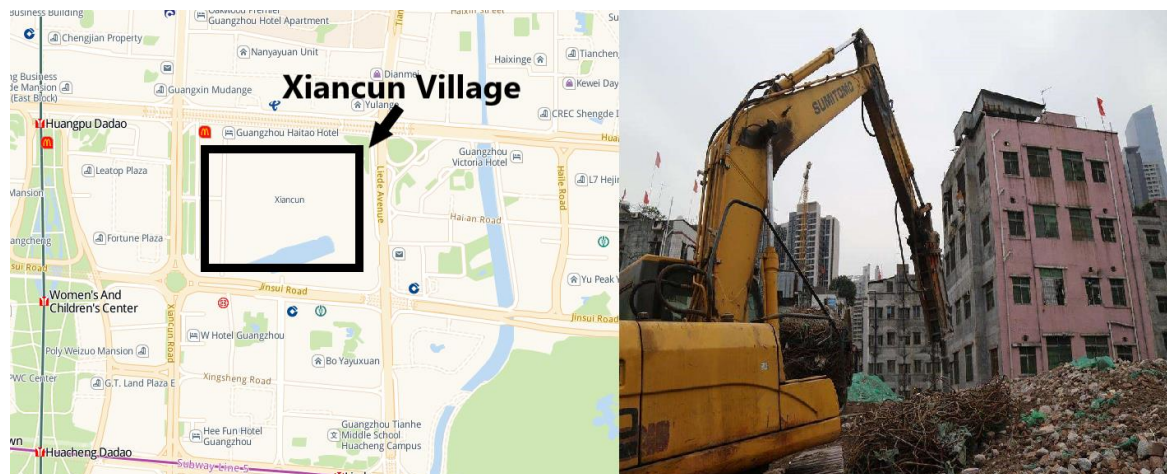
Figure 3. Xiancun old urban area reconstruction project.
