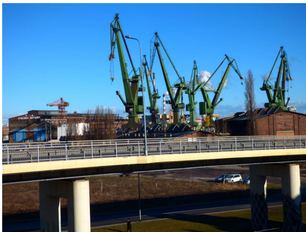
Figure 10. Newly constructed road in the former shipyard.
