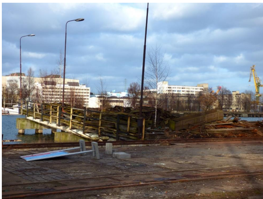
Figure 9. Ostrów Island over the canal.
