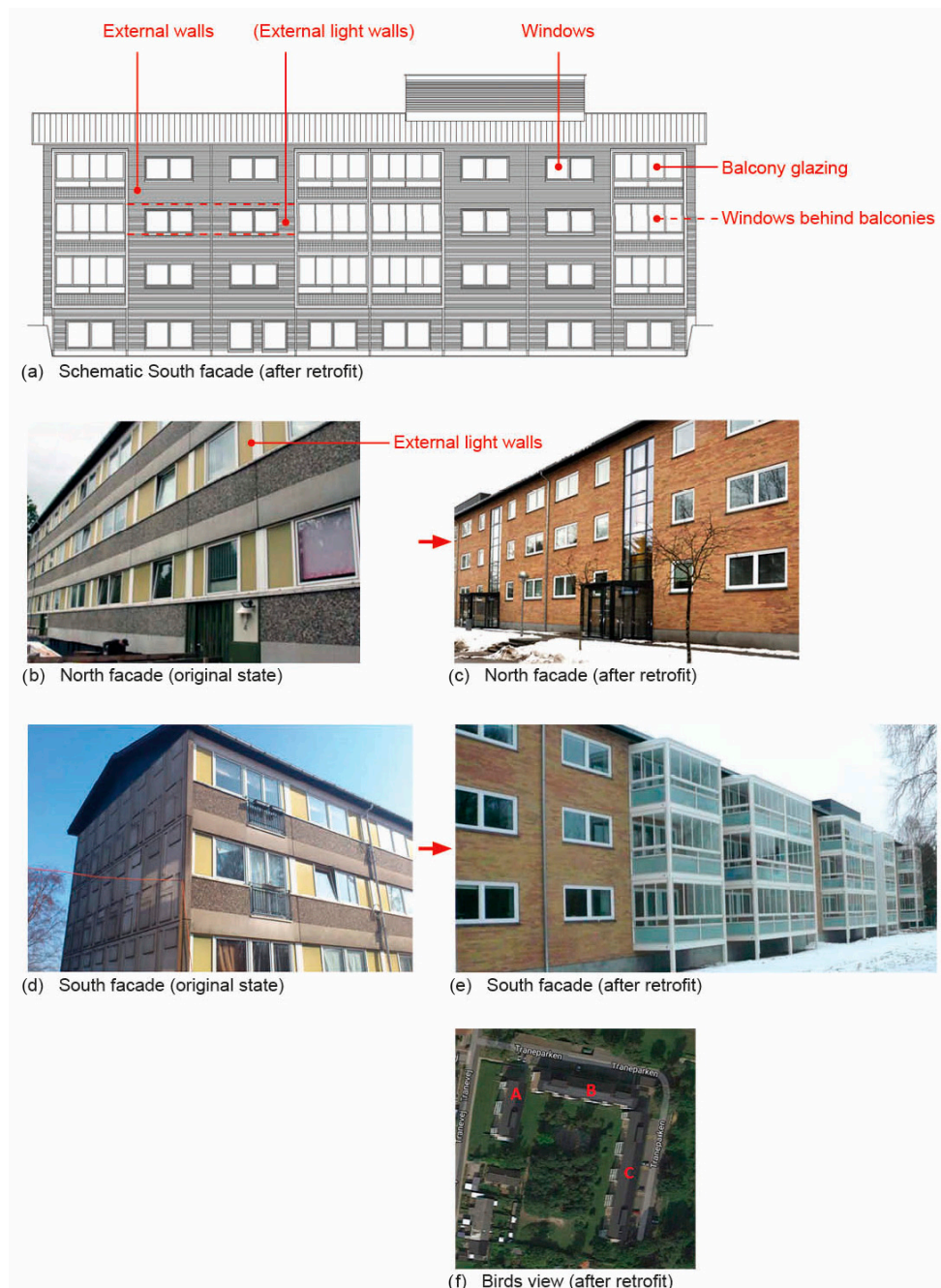
Figure 2. The social housing scheme “Traneparken” before and after the renovation.
