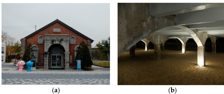
Figure 7. (a) Former pumping station, now used as the main exhibition hall of Seoul's waterworks museum. (b) Former slow sand filter beds, now a display hall in the waterworks museum. (Photo taken by the author).
