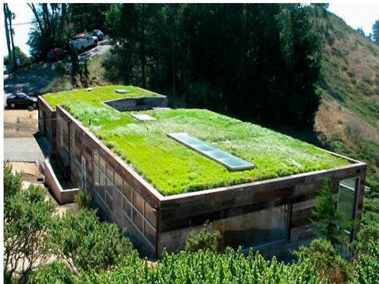
Figure 5. Extensive green roof [38].
