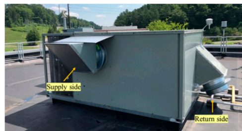
Figure 13. Damper installation for duct leakage test on supply and return sides.
